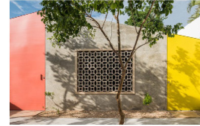
Use of stucco on the exterior, in combination with concrete lattice work , juxtaposed with brightly painted doors
